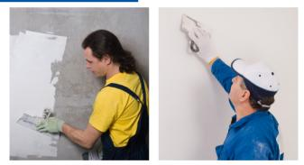
It is suitable for skimming gypsum board, sand / cement render, concrete panels and lightweight concrete surfaces.
