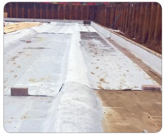
When placed below a new raft, the poured concrete engages into the locking fleece
