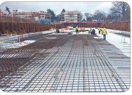
Reinforcement steel can be placed on top of the HydroBond ready for the concrete to be placed
