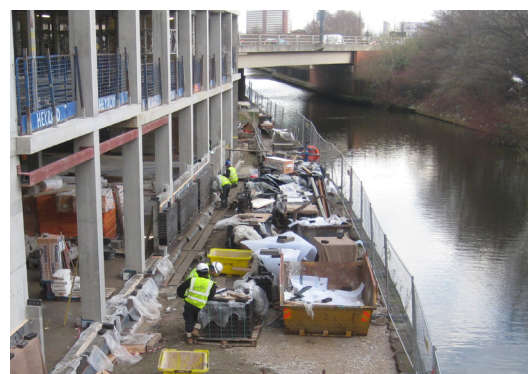
Proximity to the canal meant a robust waterproofing system was needed
