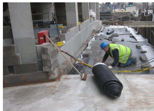
Newton 101F applied to outer face of capping beam, concrete deck and construction joints
