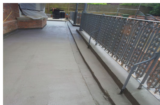
Newton Acriflex Winter applied to balcony providing a seamless waterproofing membrane
