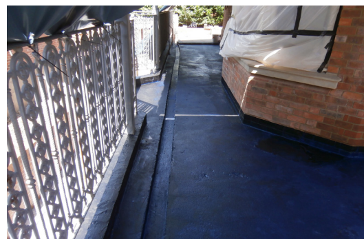
The podium deck primed with Newton NuSeal-LM
