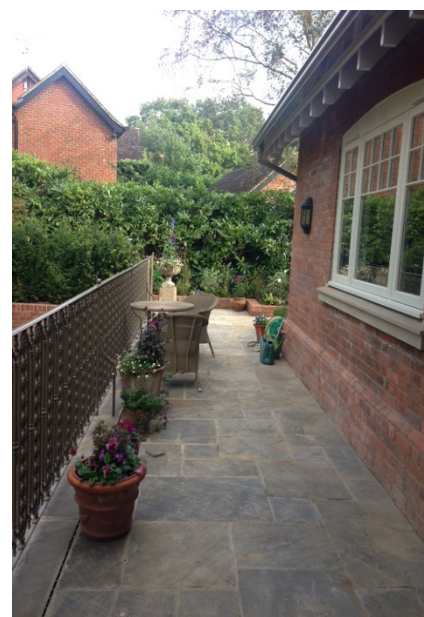
Newton Acriflex Winter applied to the finished terrace
