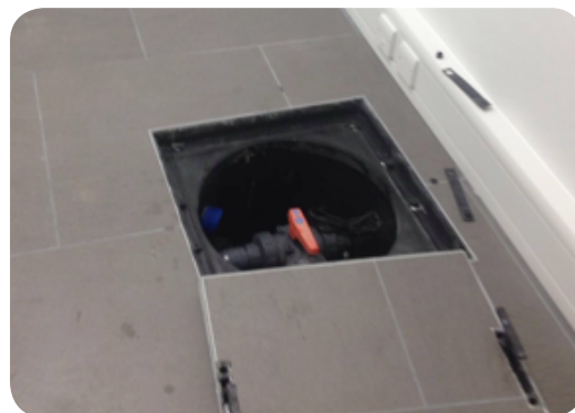
Four Titan-2 sump chambers, each with dual CP pumps provided plenty of drainage for the system
