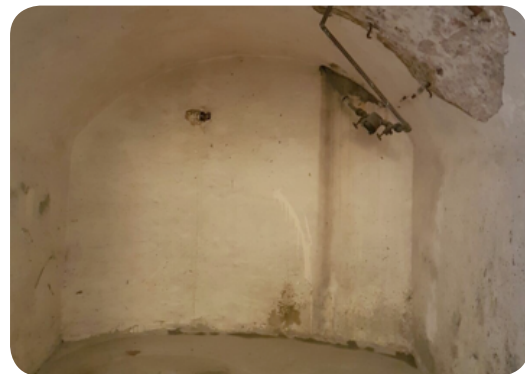
The competitor waterproof render applied internally to the vaults had failed and was allowing multiple leaks
