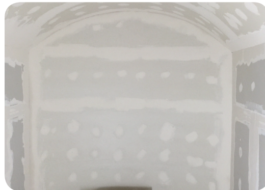
Timber battens fixed into the heads of the MultiPlugs allowed plasterboard to be applied directly over
