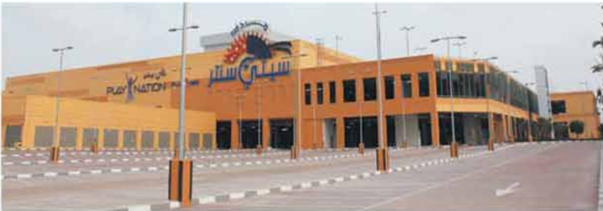
Mirdif City Center - Dubai, UAE
