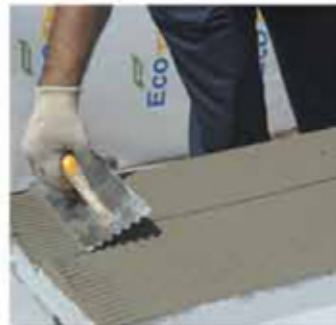
Styrofix Notched Trowel Application
