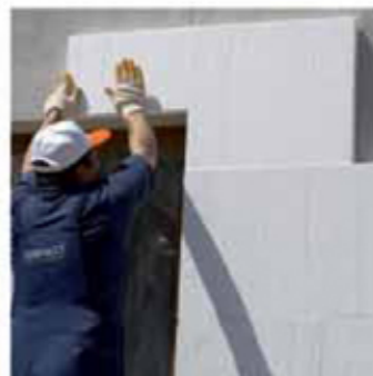
Insulation Board should never align with window corners
