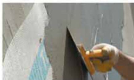
Embedding Glass Fibre Mesh
