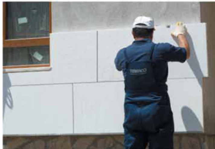
Insulation Board should never align with window corners
