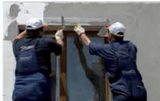
Mesh application at window edges
