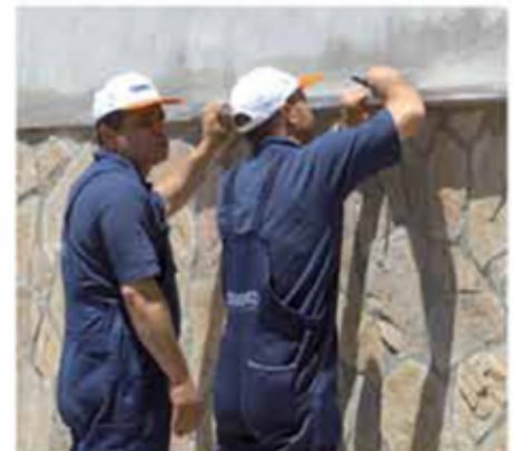
Installing Starter Base Profile
