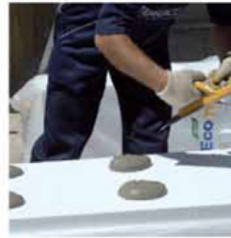
Styrofix Spot Application
