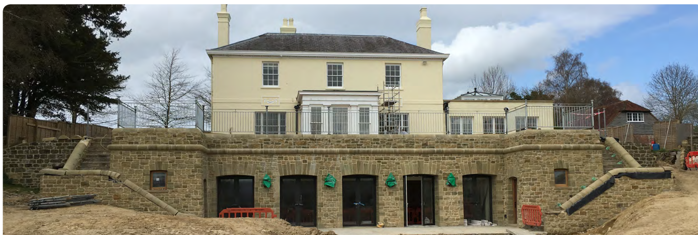
New Build Basement Pulborough, West Sussex
