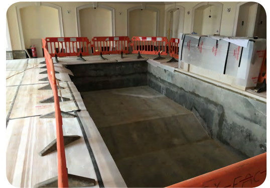
The below-ground swimming pool also required complete waterproofing with Newton products
