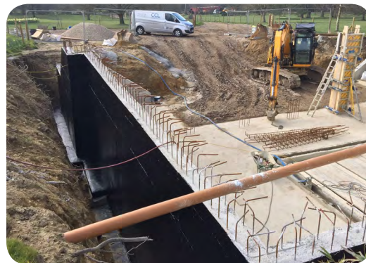
Newton 403 HydroBond and 109-LM combined to provide continuous external waterproofing protection
