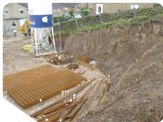
The naturally sloping site required large excavations in order to accommodate the 12 new-build properties
