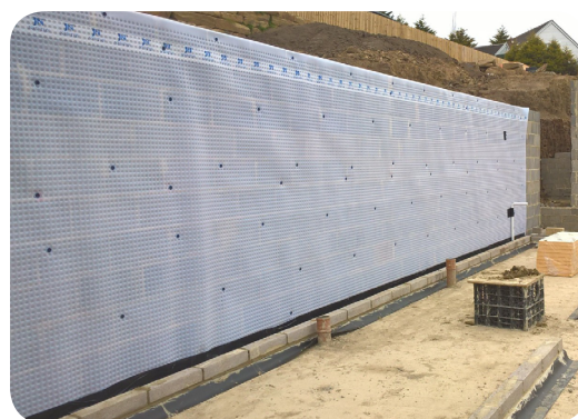
Protectahome's specialist operatives installed a neat and fully maintainable Newton CDM System
