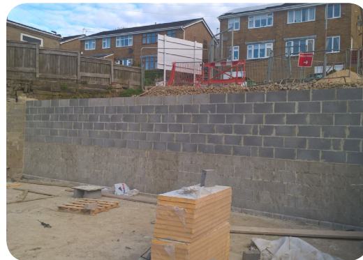
The blockwork retaining walls required both Type A external and Type C internal waterproofing protection
