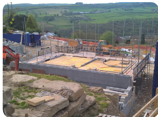
Once excavated and with the blockwork in place, the structure was ready to be waterproofed
