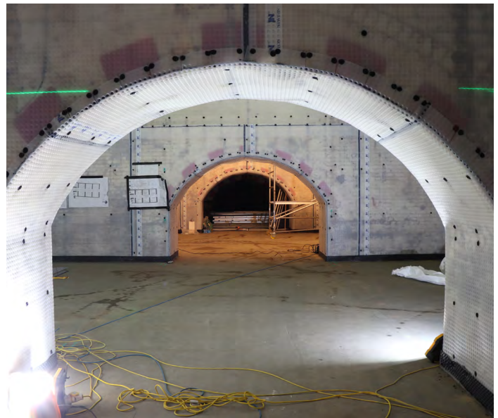
The network of vaults extends a long way beneath the streets of London.
