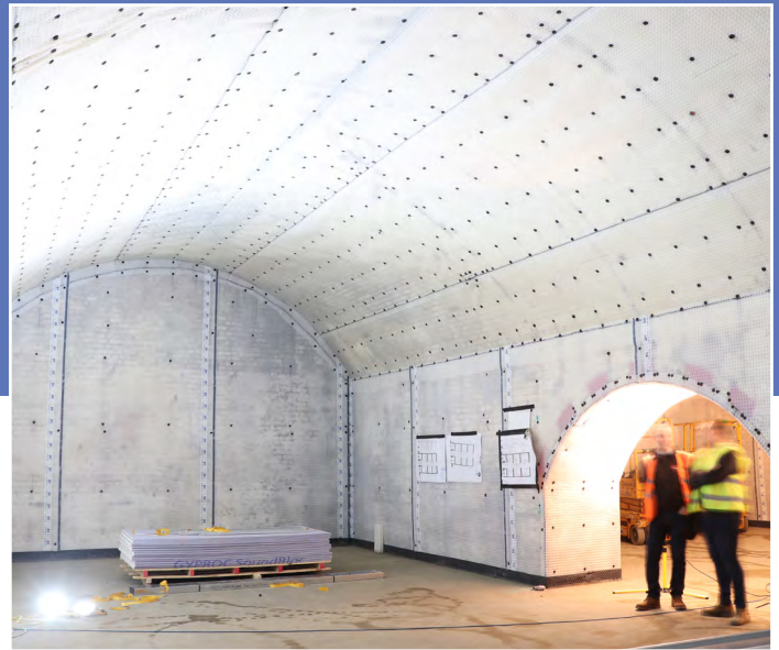
The finished cavity drain installation was exceptionally neat.
