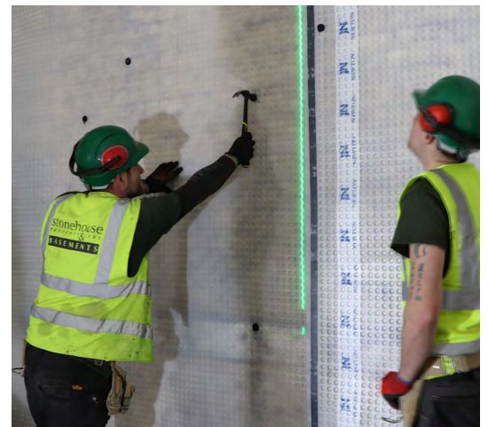
Stonehouse are experienced waterproofing installers.
