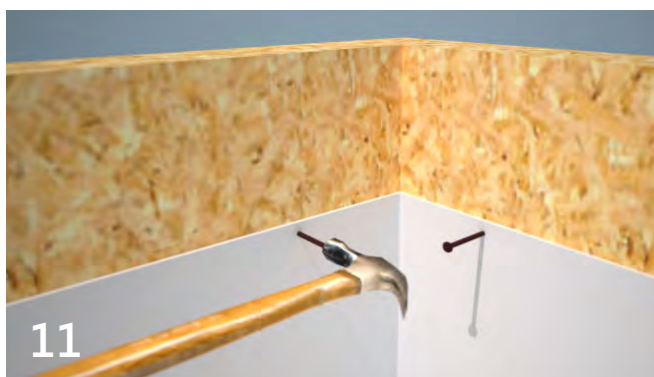
Nail the 403 HydroBond to the formwork leaving the nails exposed to give a key for the concrete and to ensure that the formwork can be easily removed. The nails are cut flush with the membrane after the formwork is removed. A dab of 106 FlexProof-X1 or 109-LM can be used over the small hole, although the membrane will self-heal.
