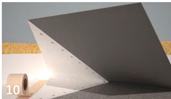
Seal the 45 degree joint with the double sided HydroBond tape. Use a hard roller to ensure a firm bond of the tape to the two surfaces of 403 HydroBond.
