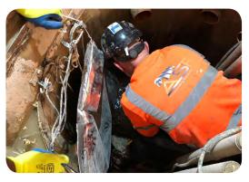
5. With the flow of water stemmed, ASF Waterproofing could now get inside the tank to inject Newton 322-SP
