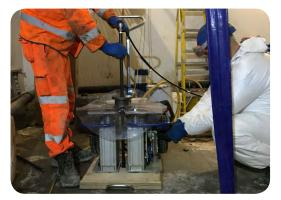
4. Once injected into the substrate, the 320-FP reacted quickly with the ground water to provide a seal
