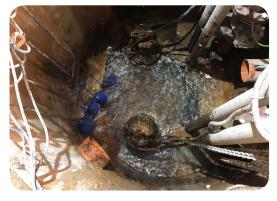
1. The cracked tank in the basement was allowing the ingress of large volumes of groundwater
