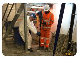
2. ASF Waterproofing first drove packers down through the slab to a depth of 2.5m around the tank
