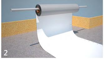
Unroll Newton 403 HydroBond with the geotextile towards the concrete to be waterproofed (white fleece facing up) using a 2m long scaffold pole or similar.
