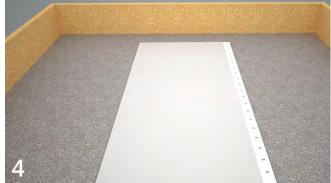
403 HydroBond is fitted to within 50mm of the top of the vertical raft temporary formwork. Mark out the height of the fold onto the membrane, marking out twice the height of the upstand, creating a guide for the fold.
