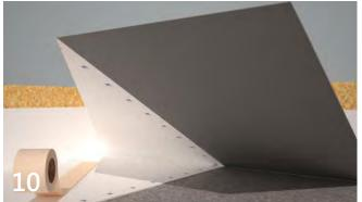
Seal the 45 degree joint with the double sided HydroBond tape. Use a hard roller to ensure a firm bond of the tape to the between the two surfaces of 403 HydroBond.
