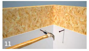
Nail the 403 HydroBond to the formwork leaving the nails exposed to give a key for the concrete and to ensure that the formwork can be easily removed. The nails are cut flush with the membrane after the formwork is removed. A dab of 106 FlexProof or 109-LM can be used over the small hole, although the membrane will self-heal.
